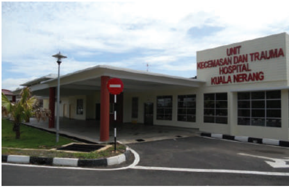
Emergency & Trauma Unit Hospital Kuala Nerang
