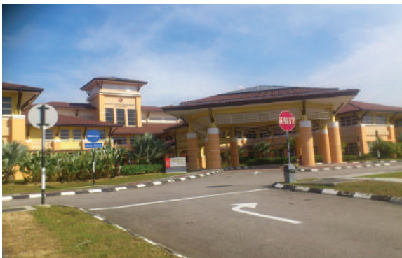
Hospital Permai, Johor
